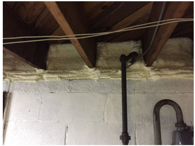
Basement Rim Joists (treated with spray foam)
