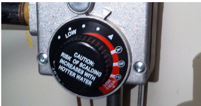
Water Heater – Temperature Control Knob
