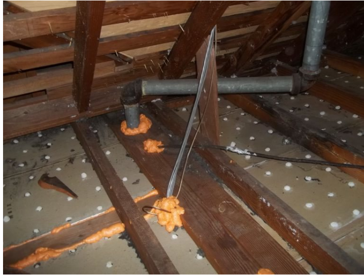
Attic Air Sealing
