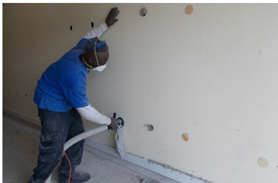
“Drill & Fill” Wall Insulation (Interior)
