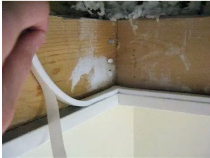
Attic Hatch Door Seal
