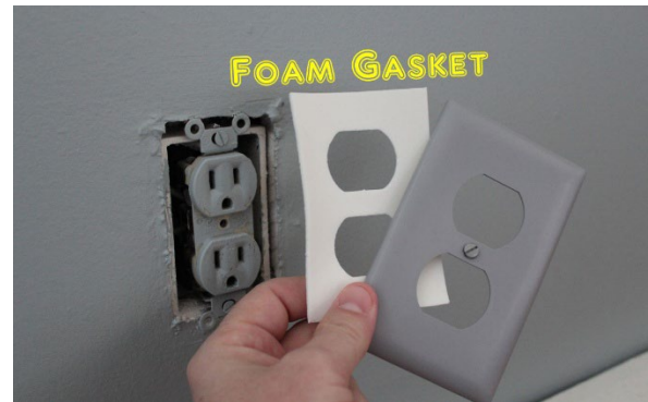
Electrical Outlet Foam Gasket
