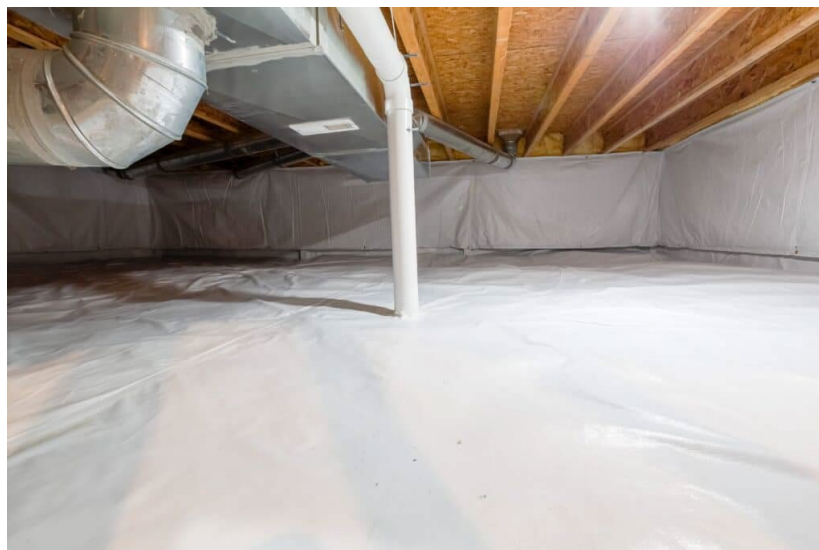
Conditioned and Encapsulated Crawl Space
