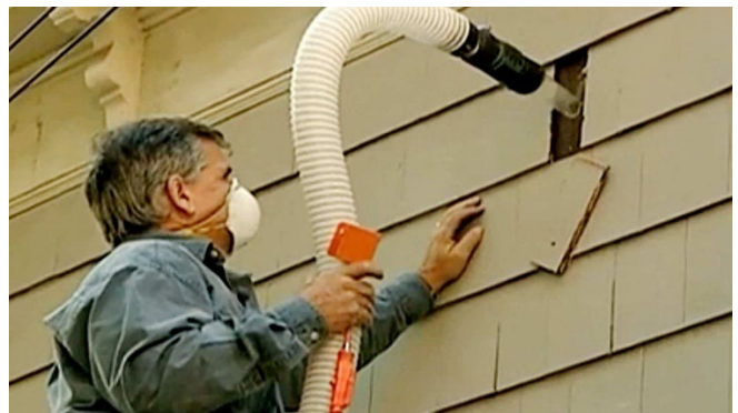
“Drill & Fill” Wall Insulation (Exterior)
