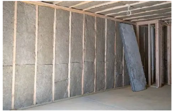
Basement Wall Insulation (Studs with Cavity Insulation, to be drywalled)
