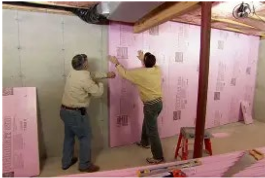
Basement Wall Insulation (Foam Board)
