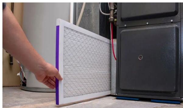
Air Filter (at Central Air Blower)
