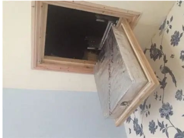
Insulated and Sealed Attic Hatch Door
