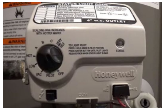
Water Heater – Temperature Control Knob
