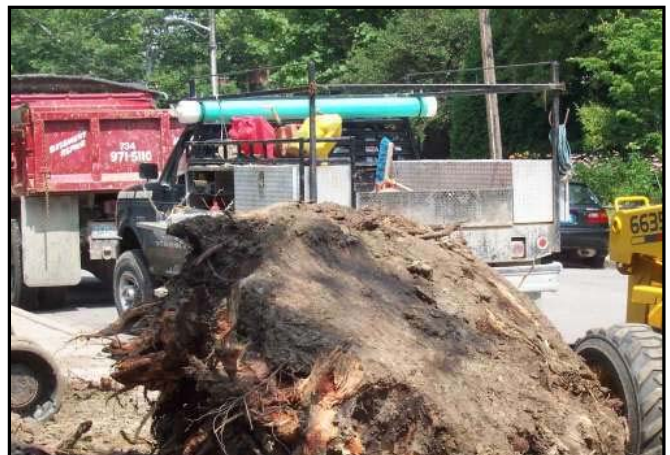
Sycamore tree root system that damaged a foundation
