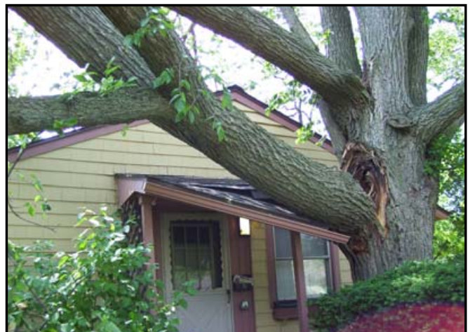
Elm tree branch that damaged the front porch
